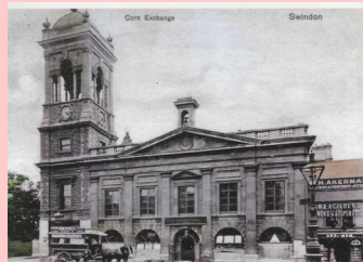
Swindon Corn Exchange, now derelict
