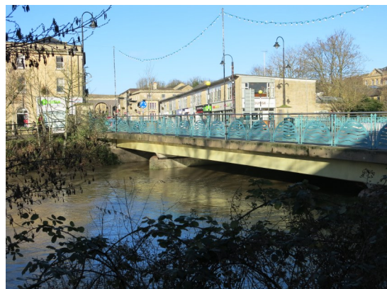
Chippenham Town Bridge today showing the 1960s concrete structure with the ‘wave’ design railings added in 2001 and designed by blacksmith Melissa Cole.
